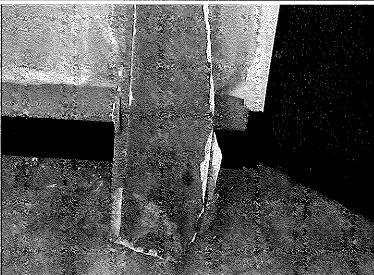
24. Conference Room 4 – View of visible mold growth on the back side of drywall removed from the north wall
