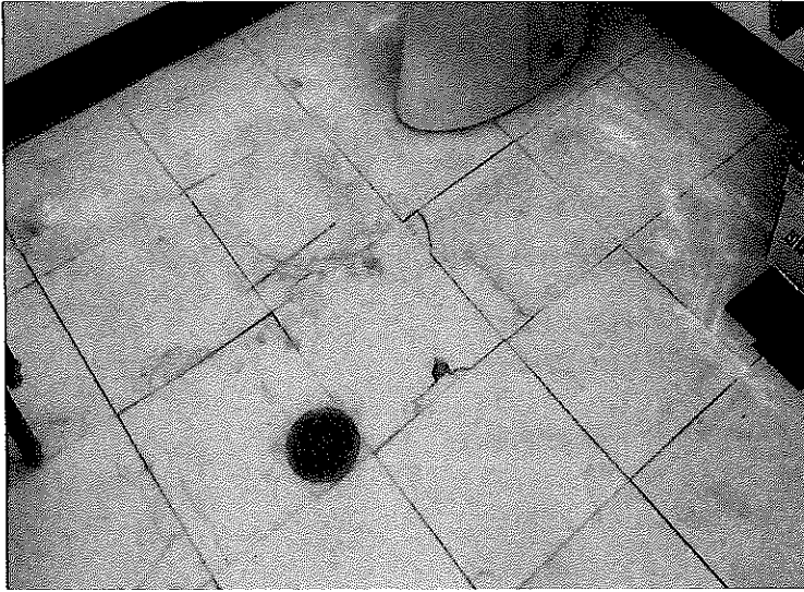
7. Asbestos Homogeneous Area 6 – White 12" x 12" floor tile with yellow adhesive; Samples 16 through 18
