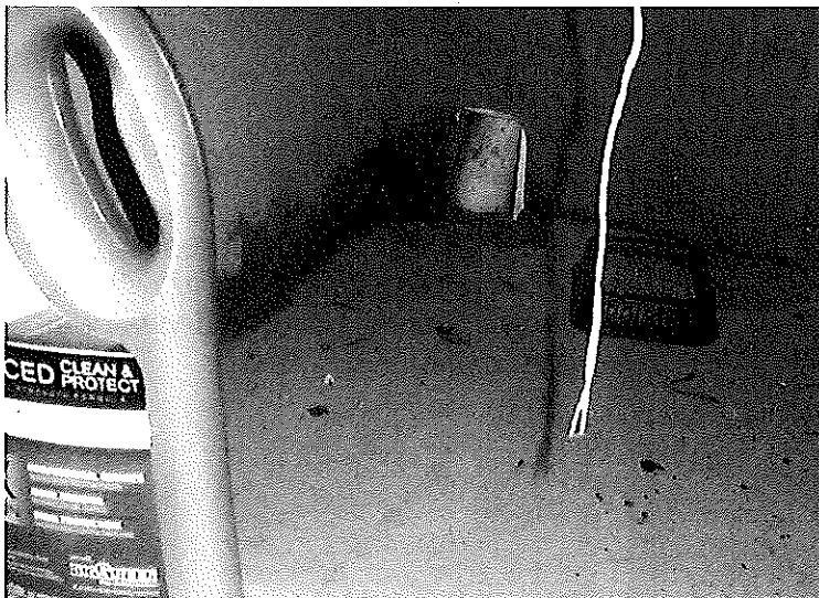
35. Break Room – View of moisture damaged surfaces within the wood sink cabinet
