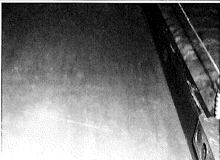
30. Hall south of Conference Room 2 – View of visible mold growth on the upper north drywall wall above ceiling tiles
