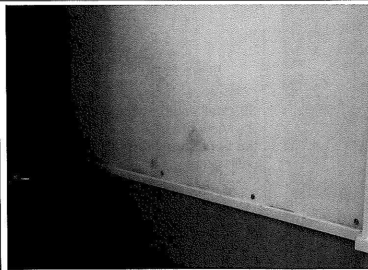
27. Conference Room 4 – View of visible mold growth on wall surfaces behind plexiglass panels
