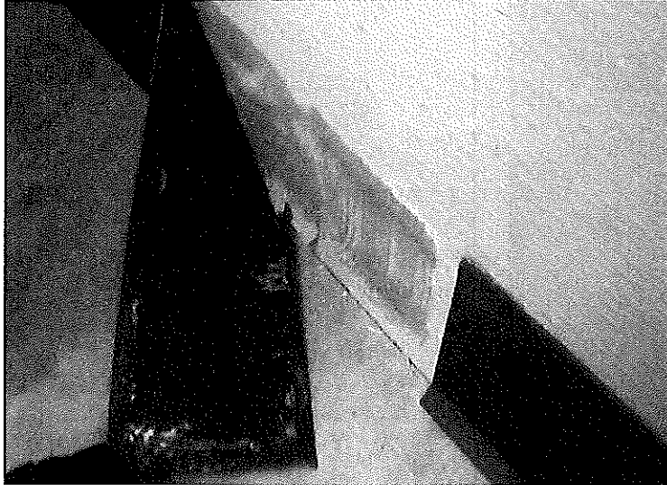
4. Asbestos Homogeneous Area 3 – Tan adhesive for vinyl cove base; Samples 07 through 09
