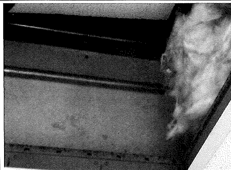
39. Hall south of the Break Room – View of visible mold growth on the upper north vinyl-covered drywall wall above ceiling tiles
