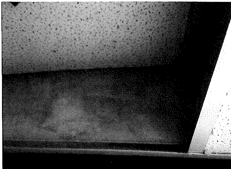
31. Hall east of Conference Room 2 – View of visible mold growth on the upper east vinyl-covered drywall wall above ceiling tiles
